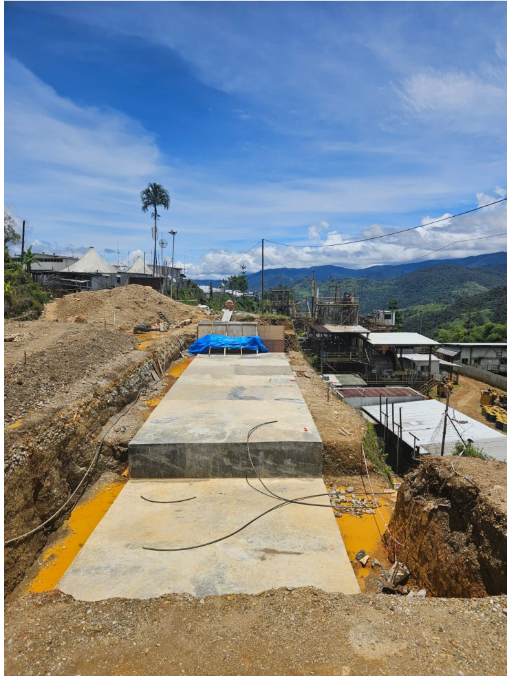
Foundations for the new APT crushing and milling circuit
