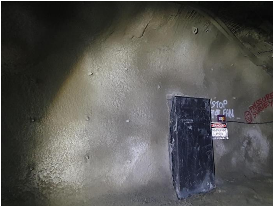
Figure 5: Vent door closing off ventilation recirculation, set in shotcrete and cable bolts for additional ground support.
