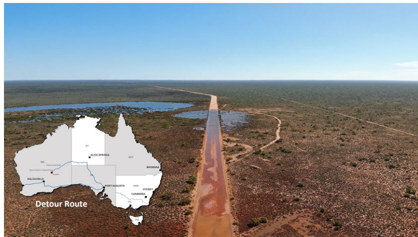
Great Central Road - 20 March 2024
