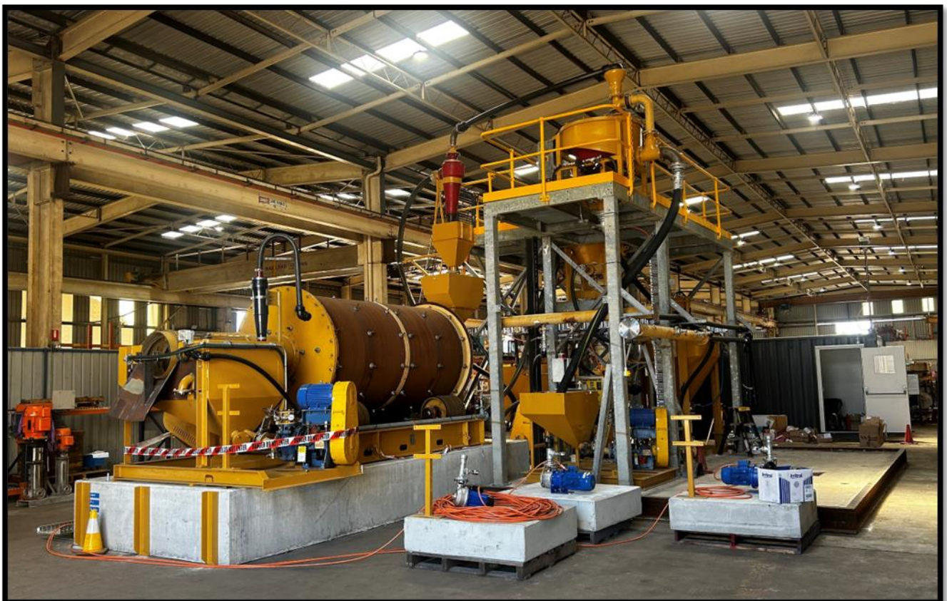
Figure 1: Gekko processing plant final overhaul before disassembling
