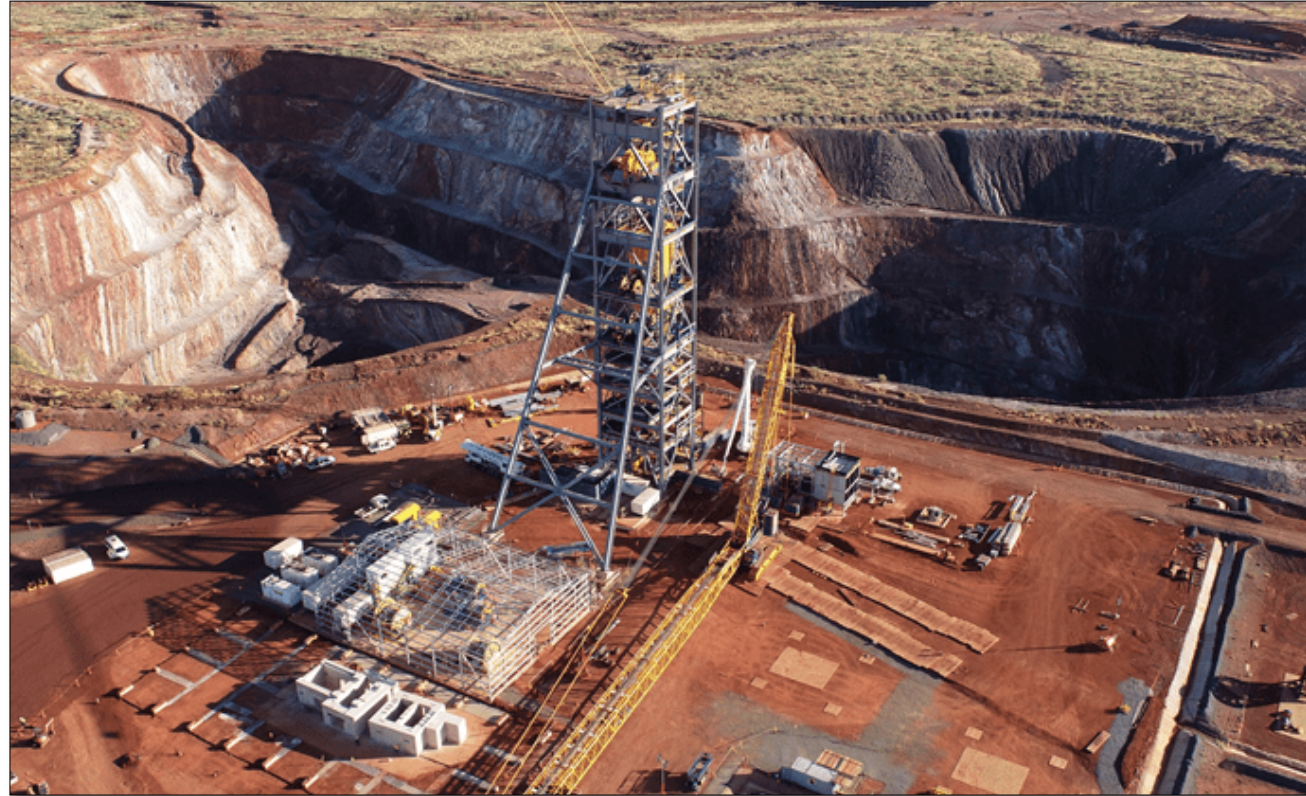
TE2 Headframe – Newmont's Tanami Gold Operations
