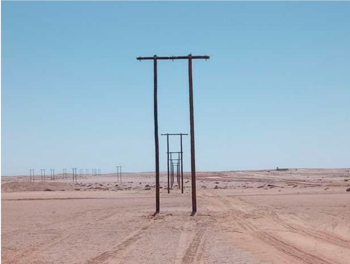
Figure 2: 33kV powerlines H-pole support structures being installed
