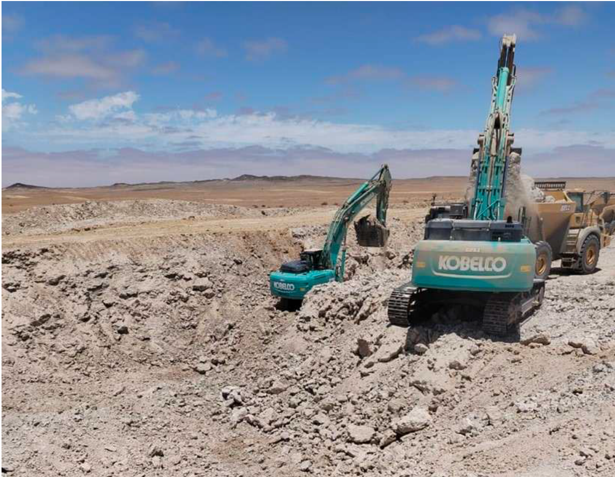
Figure 4: Excavation of primary box cut post blasting
