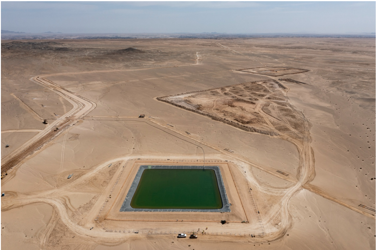
Figure 1: Completed construction water storage dam
