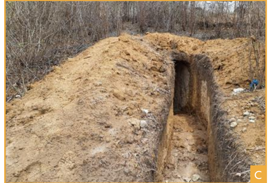
Photographic example of workings located within the larger Caraíbas tenement area (805118mE, 8193908mN) Three rock chip samples were taken from the site with peak assay results of 0.53% \text{Li}_2\text{O} , 1,245 ppm tantalum, 1,175 ppm rubidium and 1,455 ppm caesium
