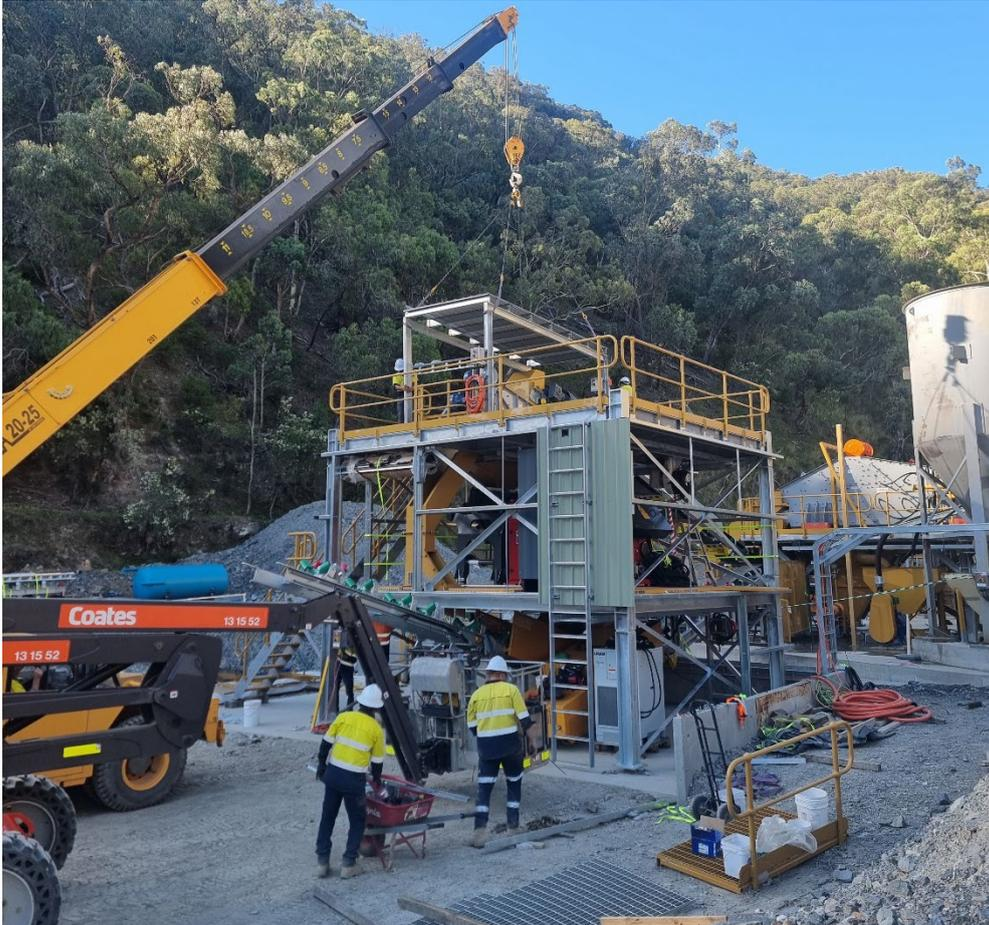
**Figure 9 Ore sorter installation well underway**
