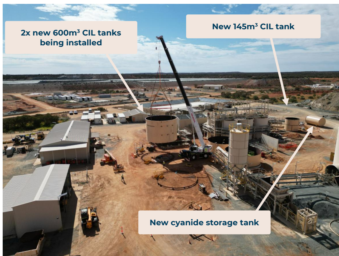
Figure 3: The 2x new 600m 3 tanks being installed for the expanded CIL circuit, December 2024.
