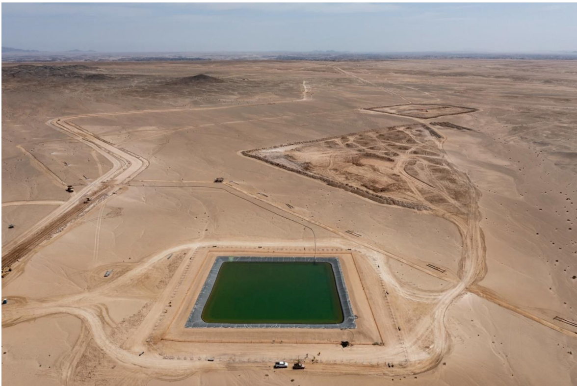
Figure 1: Completed construction water storage dam
