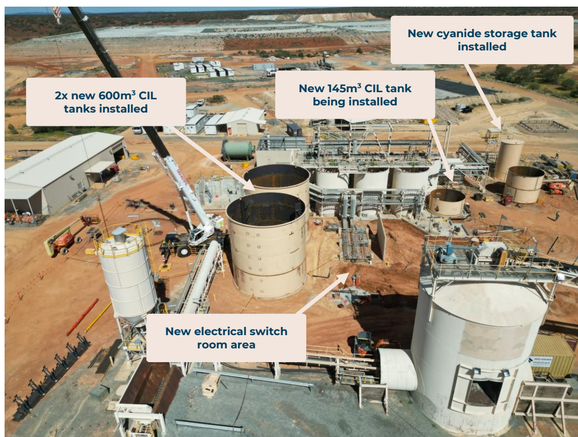
Figure 4: Progress on the expanded processing plant, January 2025.
