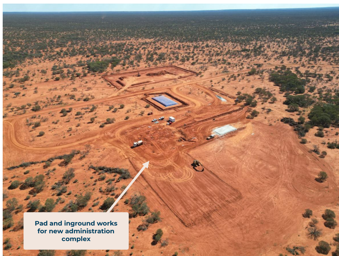
Figure 6: Civil works underway for the new Turnberry administration complex to accommodate open pit and underground operations, January 2025.
