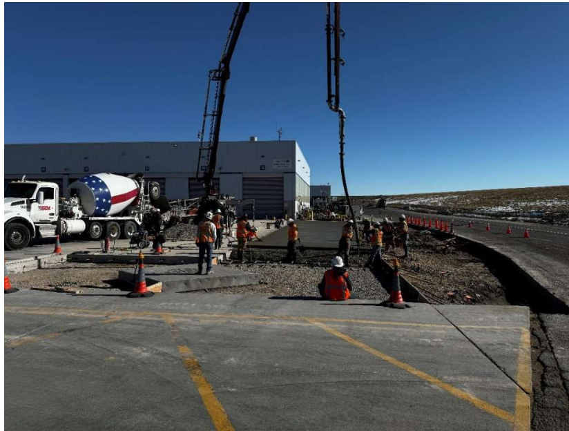
Figure 5. Replacing panes for United Airlines at Denver International Airport
