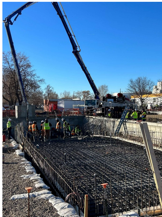
Figure 8. Installing pool flooring- City of Denver- Swansea Community Pool
