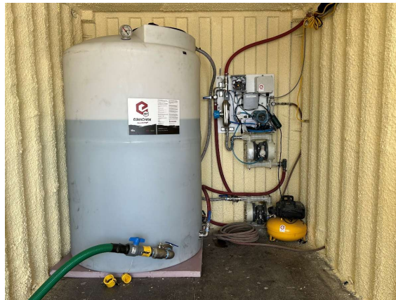
Figure 2 Holcim Broomfield Colorado Plant - 550-gallon tank, recirculation system and static wall dispenser
