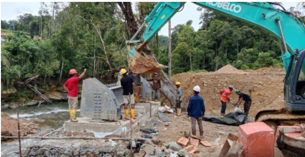
Installing steel bridge abutment A2 deck frame on 22 nd December 2024
