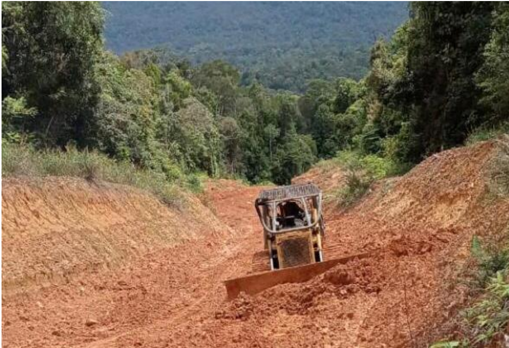
Removing soft material at KM 91
