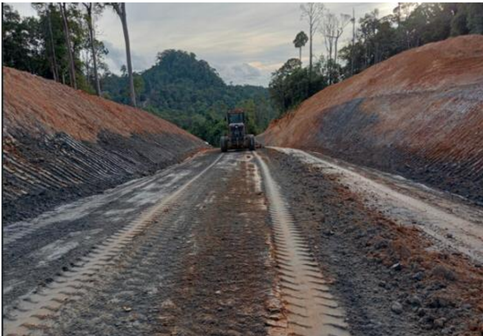
Road grading and compacting works at KM 77
