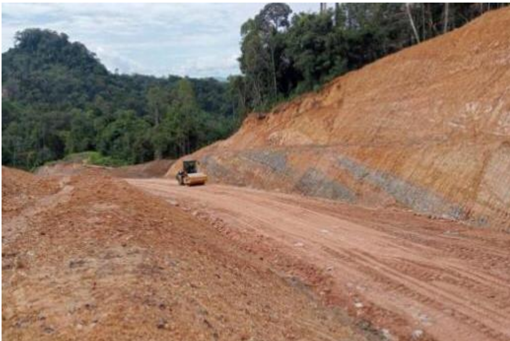
Road compaction from km 77 to km 79
