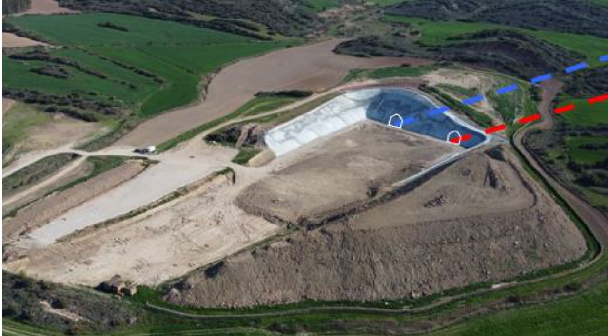
Figure 3-7: Current Status of the Surface Boxcut
