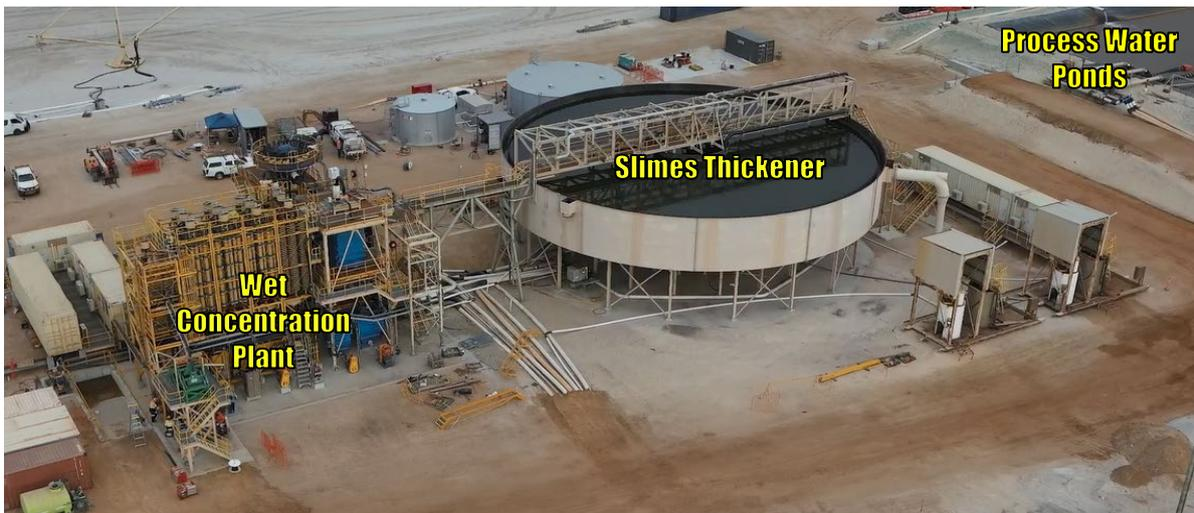
*Note: Small footprint of wet concentration plant is a result of first commercial application of Mineral Technologies CT-1 spiral technology.*
