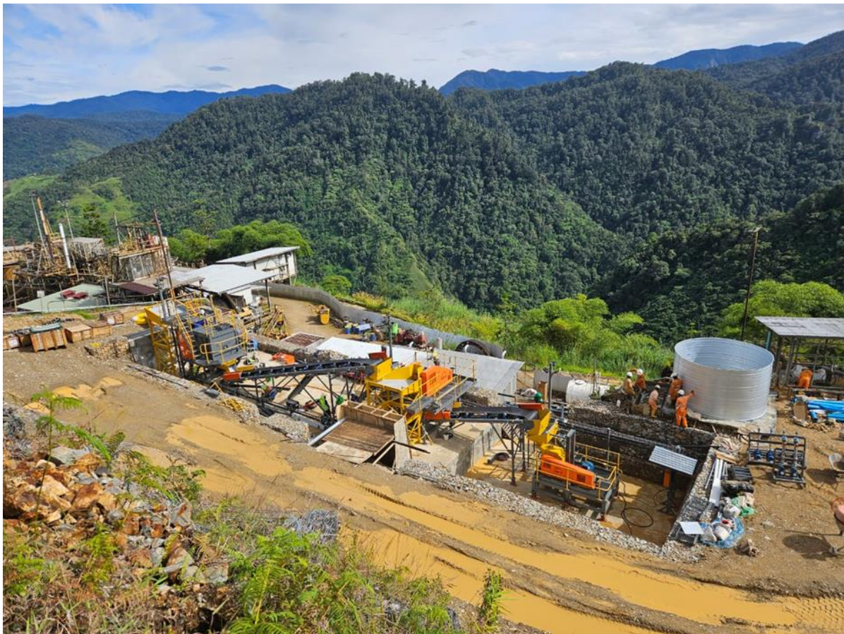
Photo 1: Modular Plant during Construction
