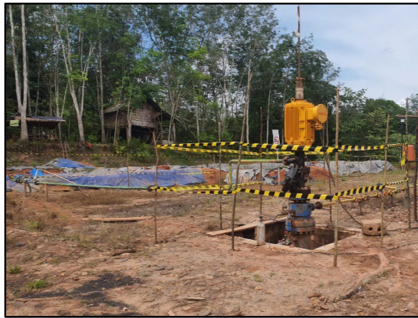
Dewatering Process in MU-005 TW
