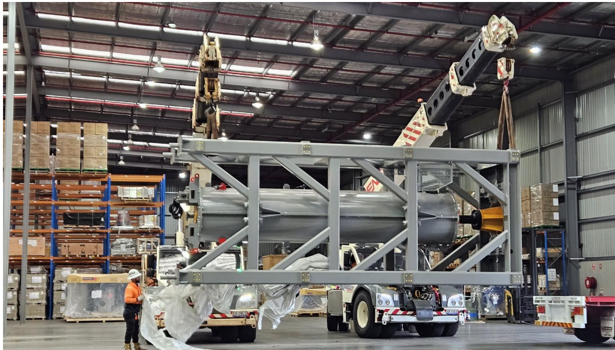
SAG mill main assembly
