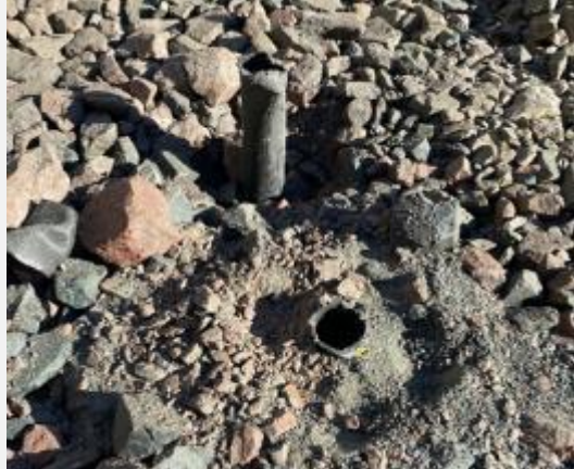
TRADITIONAL PIPING PROCESS WITH POOR BLAST OUTCOMES
