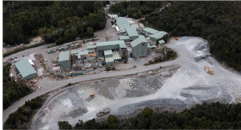
300ktpa CIL Plant & Administration Complex
