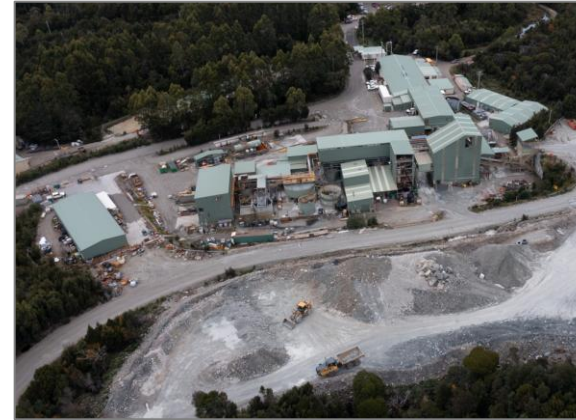
300ktpa CIL Plant & Administration Complex
