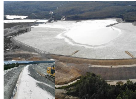
Henty TSF and Jan 2025 works (inset)
