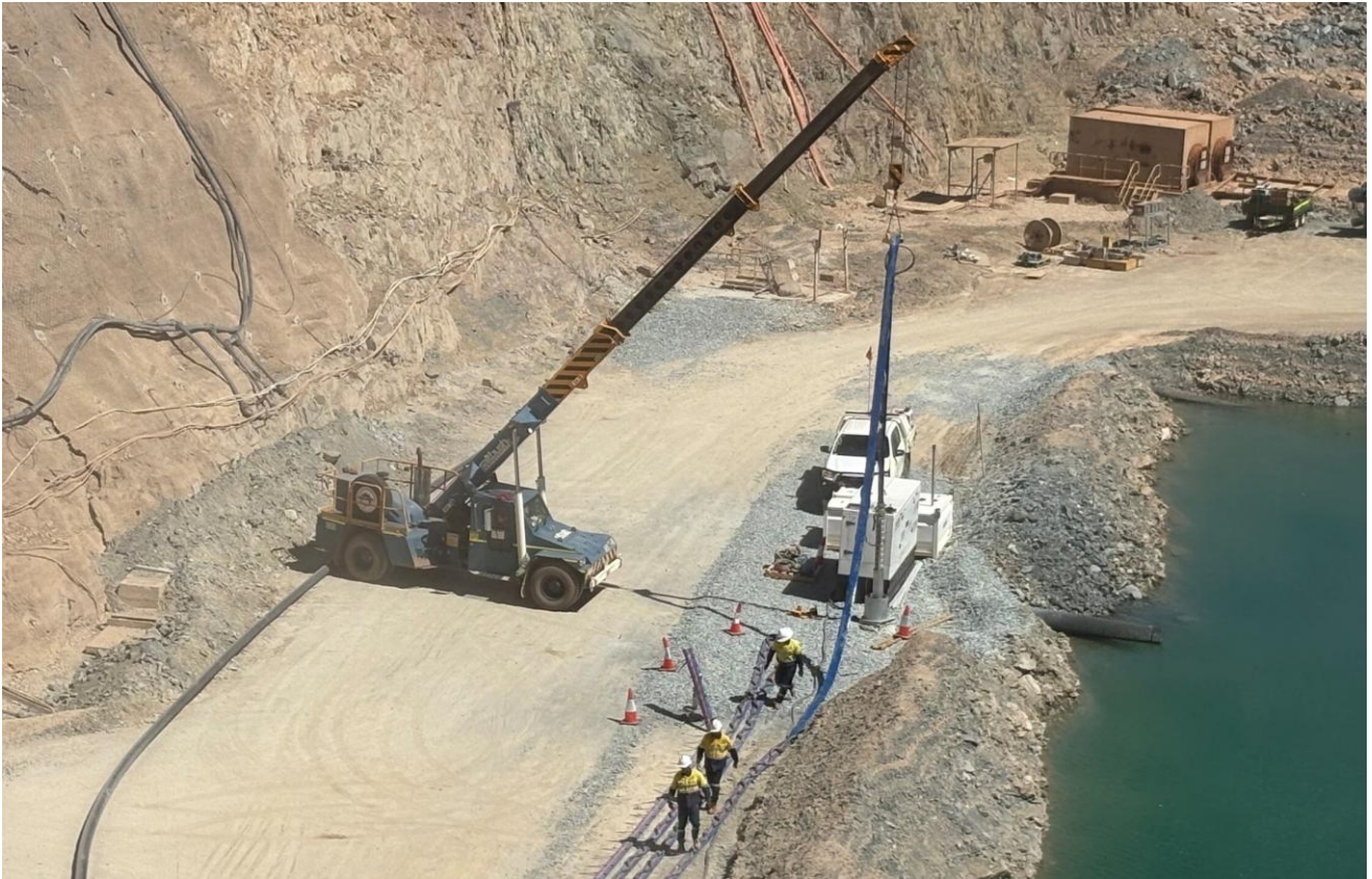
Figure 8: Installation of dewatering pump down a 12 inch bore hole drilled at the base of the Wilber open pit into the underground workings at the high-grade Andy Well underground mine, March 2025.
