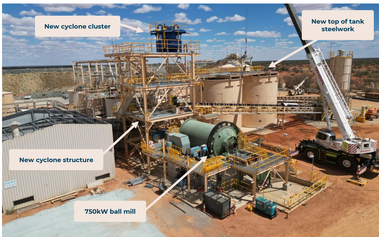
Figure 2: The larger 750kW ball mill, cyclone cluster and top of tank steel work installed, March 2025.
