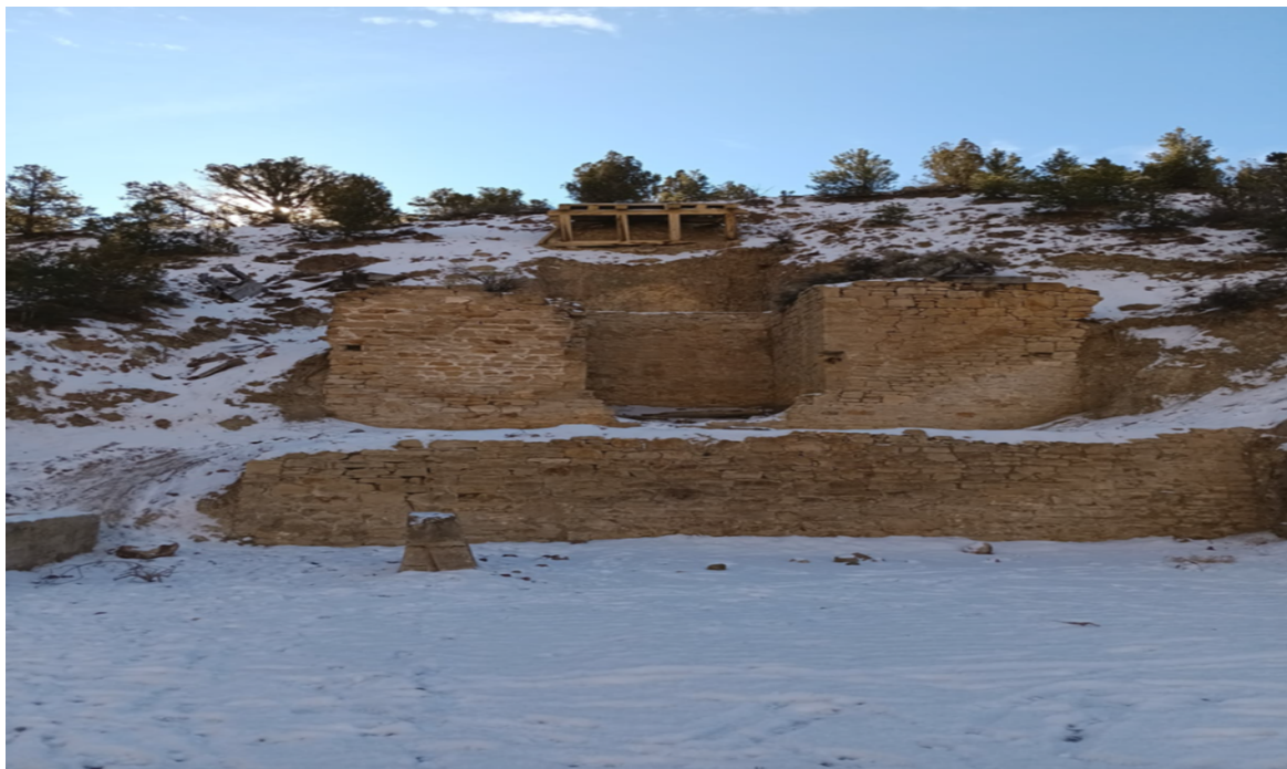
Photo 3. Old Mill site at Coyote Creek
