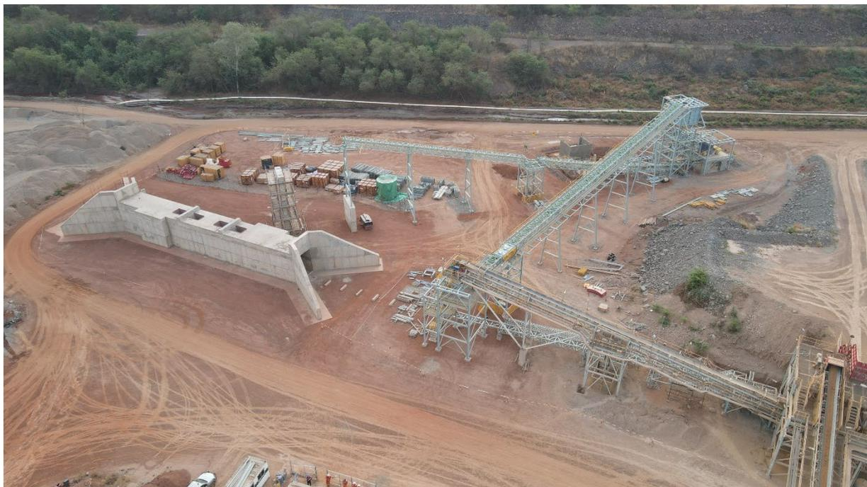
**Figure 11: Secondary crusher and sulphide stockpile feed conveyor areas are 50% and 30% complete respectively**
