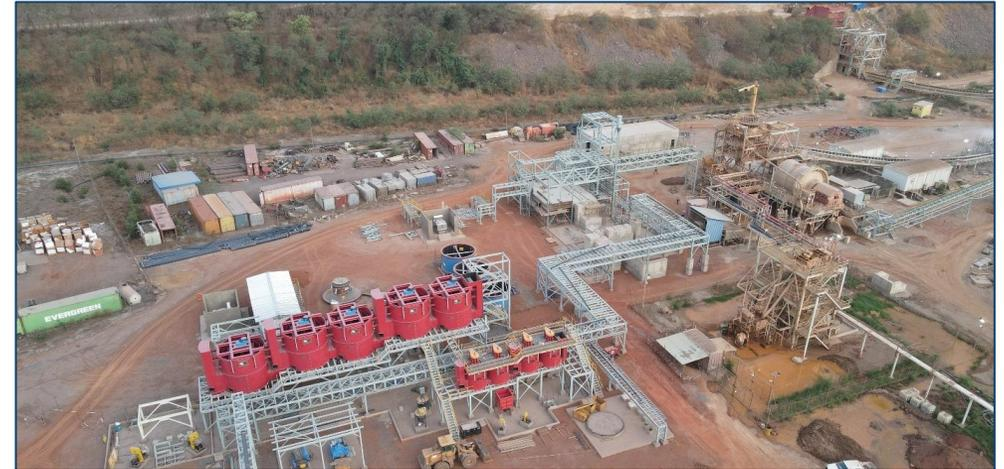
Ball mill and flotation areas under construction. The flotation circuit is now 86% complete, while the ball mill areas is 35% complete
