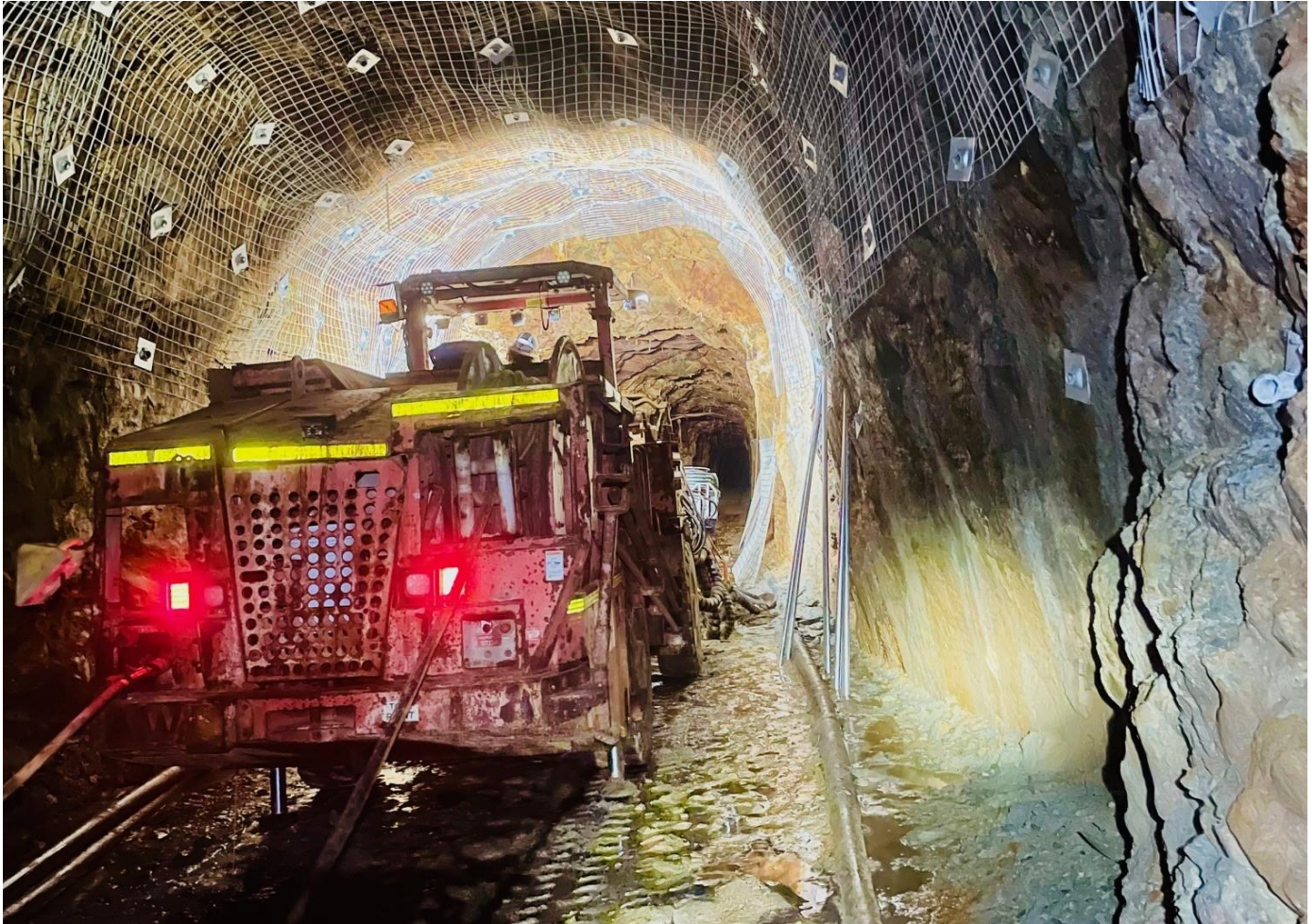
Figure 5: Installation of ground support in the Southern Ore Zone at Mineral Hill.
