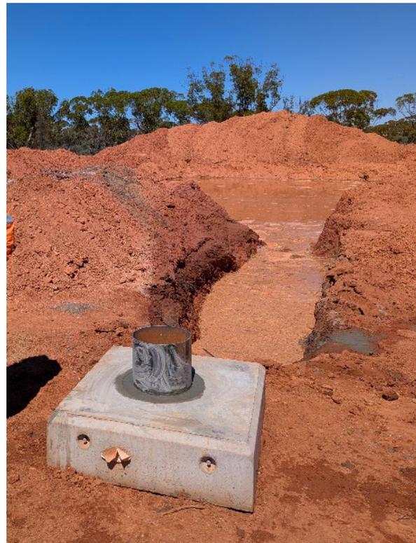
Figure 9: Test pumping well completed at Goongarrie Hub
