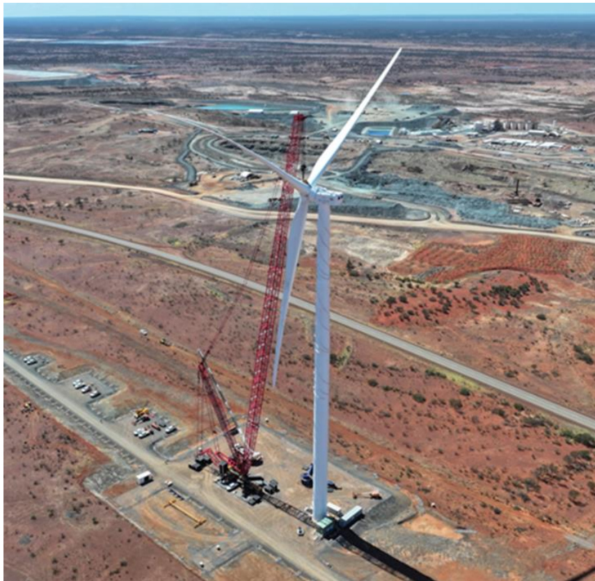
Figure 12: 6MW wind turbine installation, to be completed by H2 FY25.
