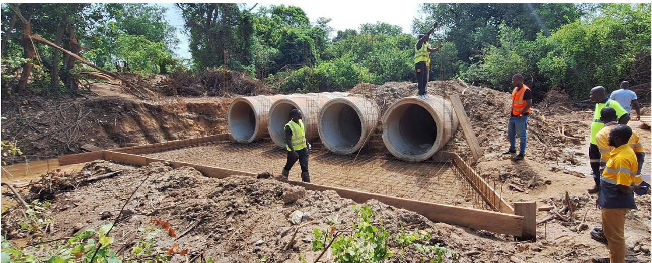
*Figure 7: Construction in progress of a bridge between Napié's two existing gold deposits*
