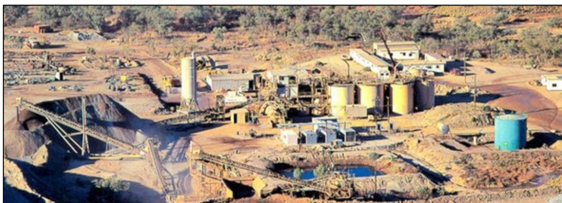
Figure 3: Butchers Creek gold processing plant. Circa 1996.
