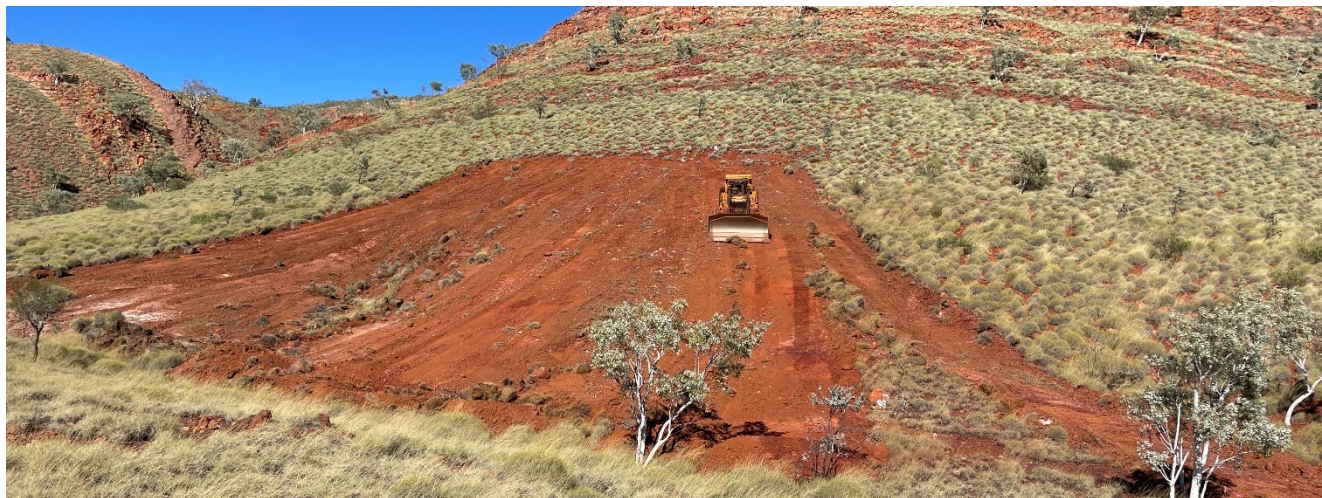
Figure 5: Clearing of the Boxcut oxide layer and clearing of the mine infrastructure and process plant footprint.
