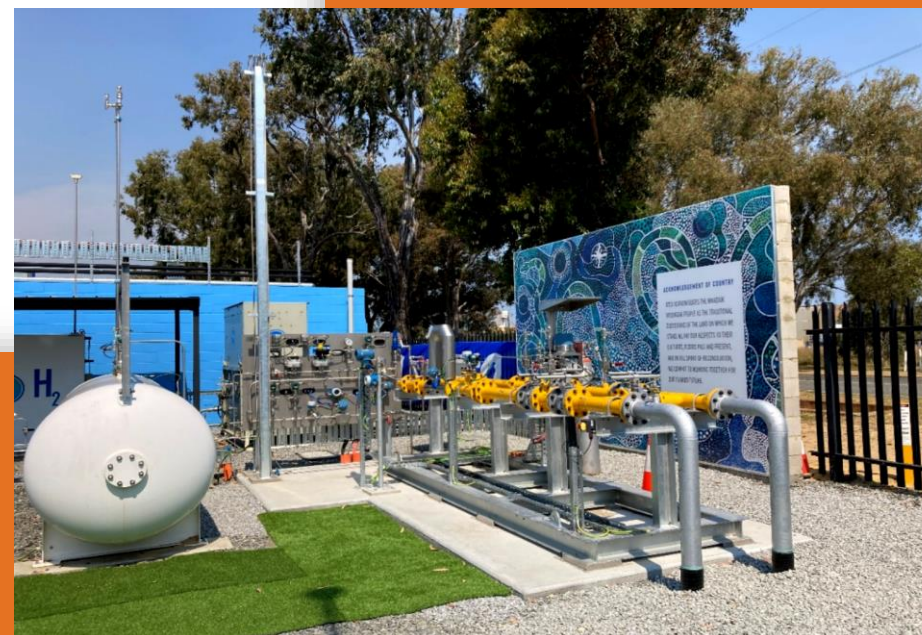
ATCO's fully commissioned H 2 Blending Station at Jandakot
