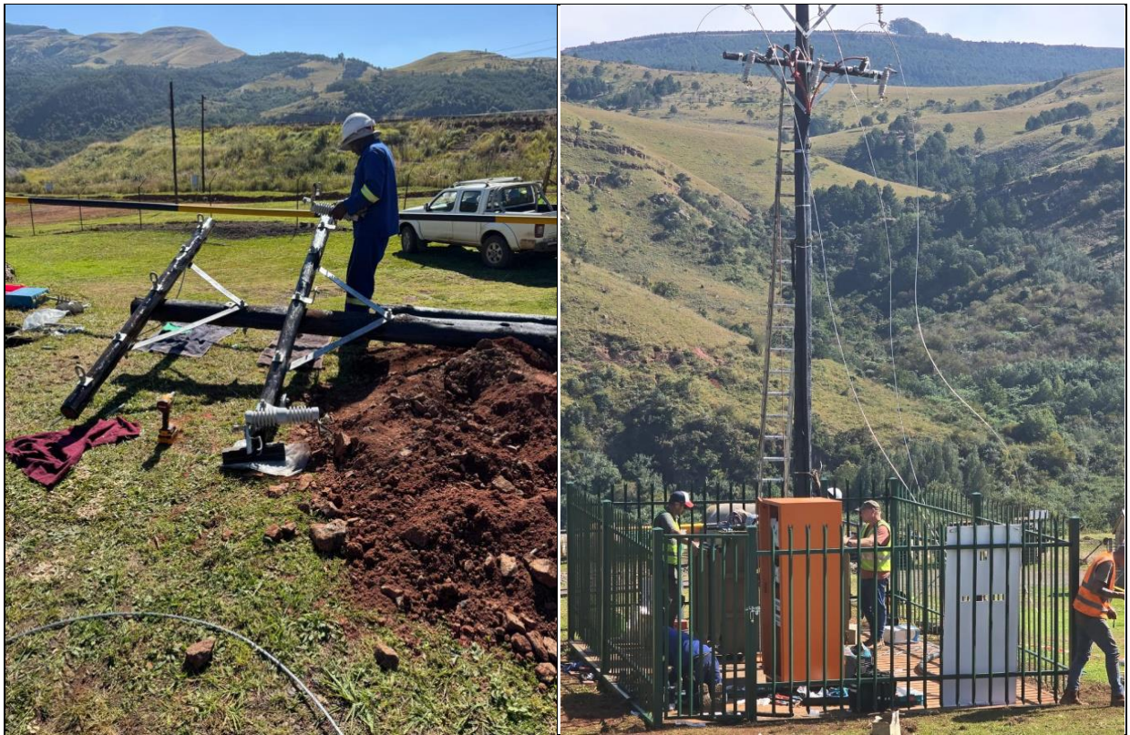
Figure 3: Installation of temporary electrical plant supply
