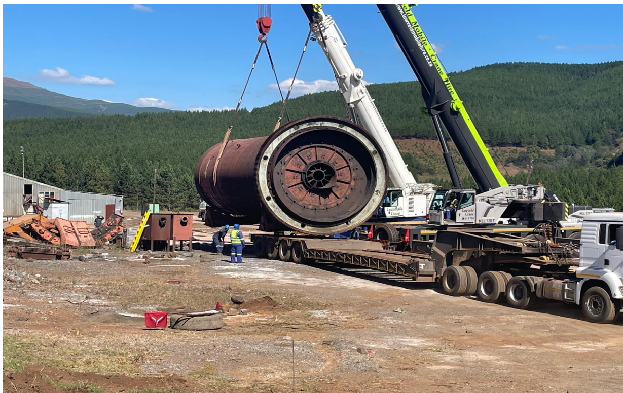
Figure 5: Lifting and loading of the big ball mill for transport to the laydown area
