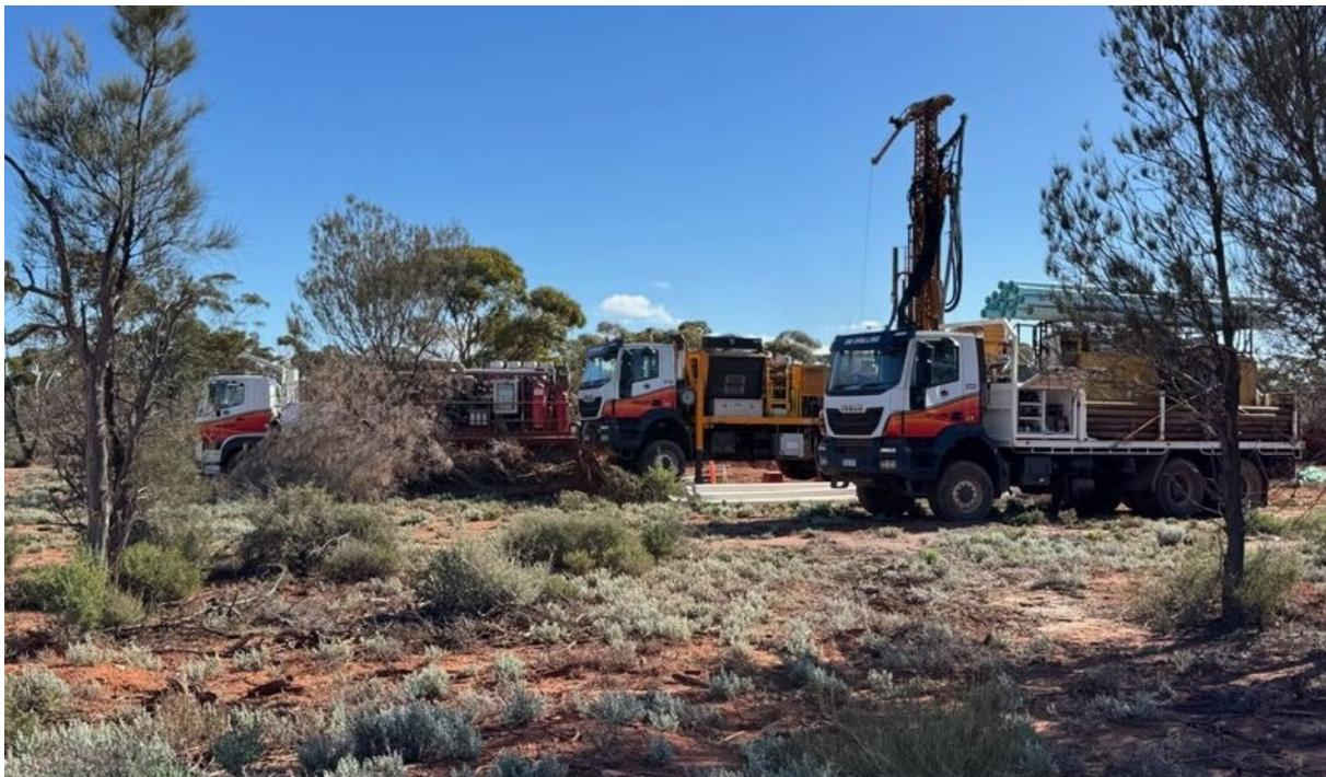
*Figure 3: Second RC Drill Rig on site completing pump test holes supporting hydrogeological studies*
