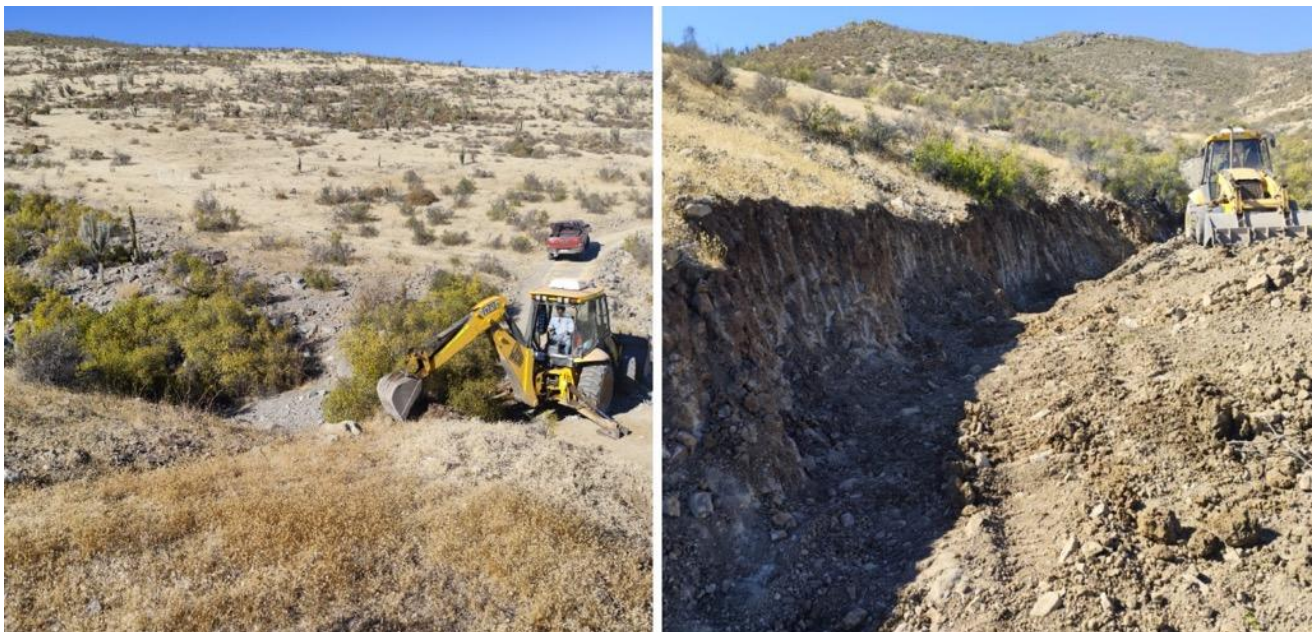
Figure 6: Backhoe preparing drill pad (left) and excavating trench 7 in the northern sector of La Florida Prospect.
