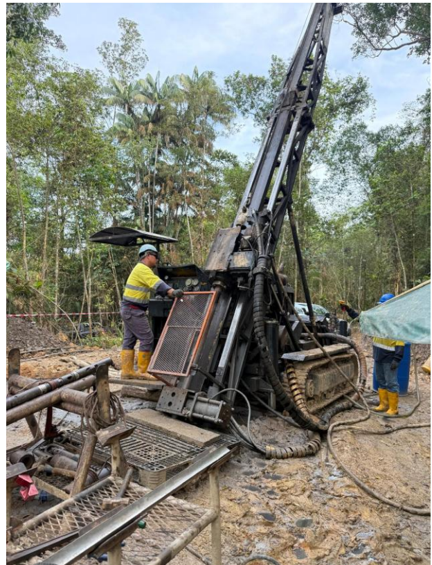
Rig 76 and Rig 38 on their final 300 metre holes for the 1,720 metre geotechnical drilling programme.
