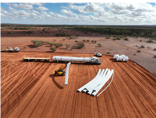
Figure 2 – Water pipeline being unloaded
