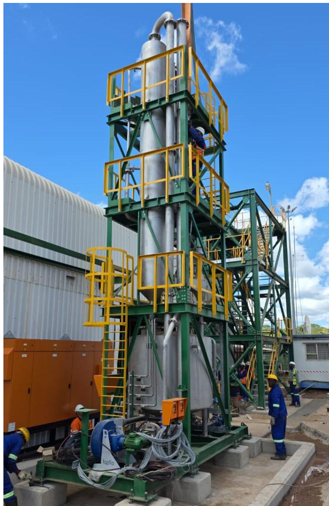
Figure 6: Placement of the new off-gas scrubber outside the drying and packaging building
