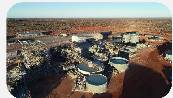
Aerial view of plant
