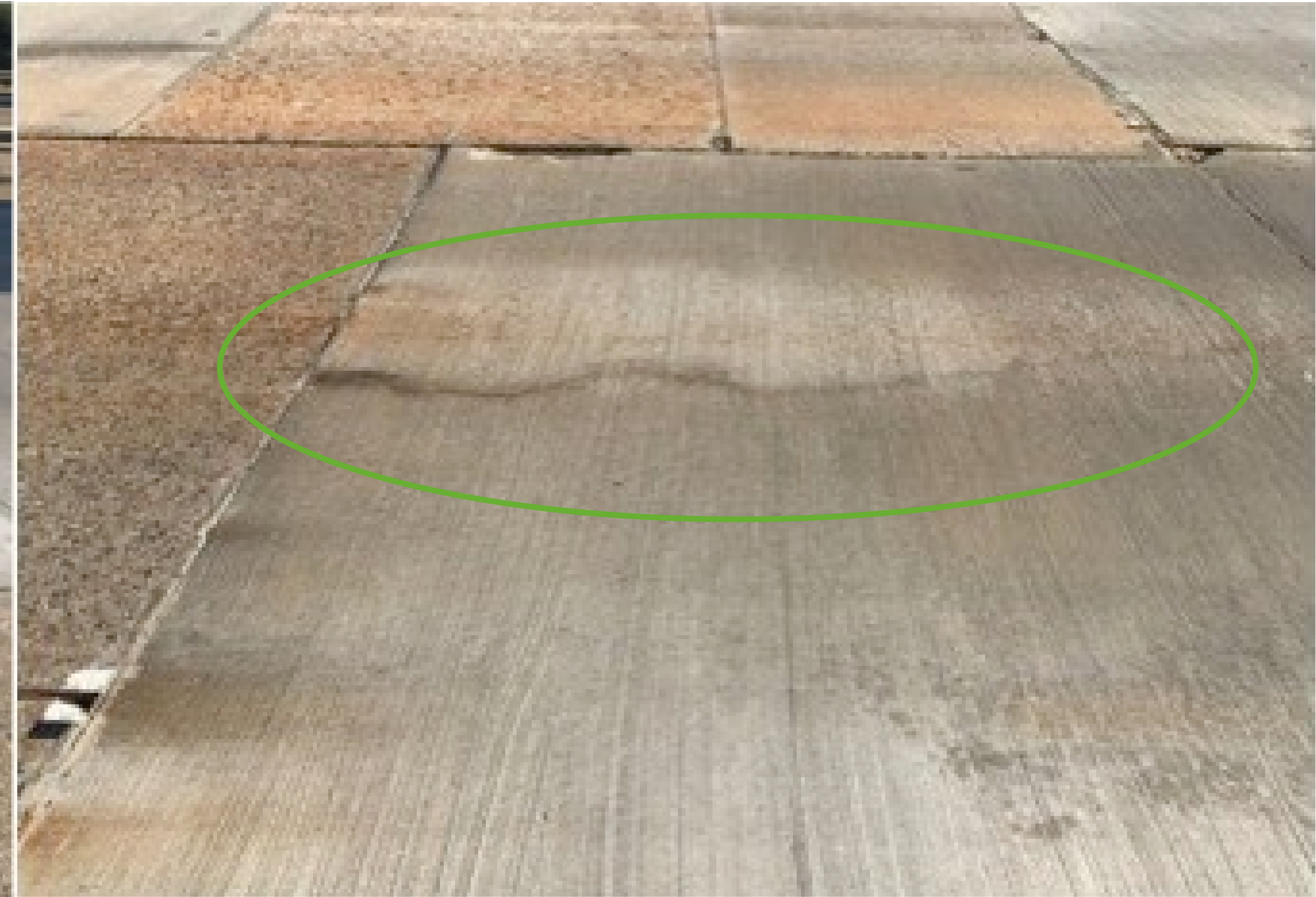
Control – Visible cracking and Wear
