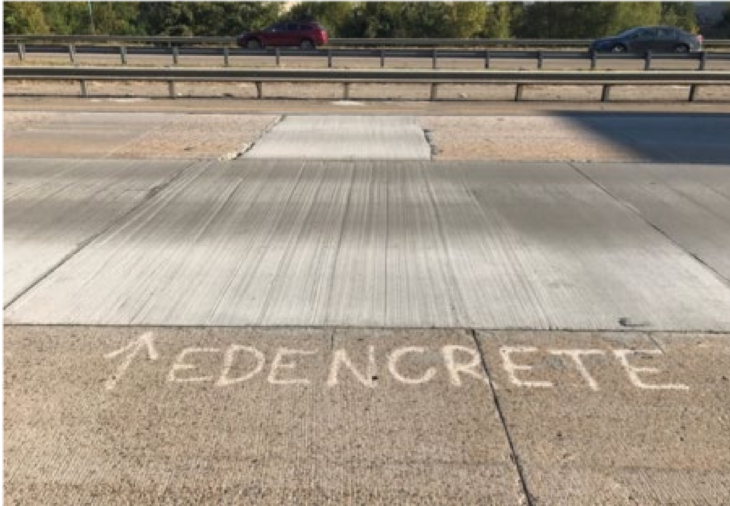
EdenCrete® – No visible cracking or wear
