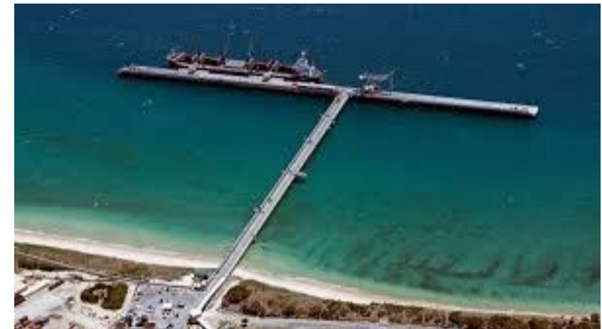
Open pile jetty with conveyor system
