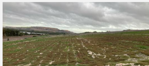
Peak Downs Rehabilitation Works
