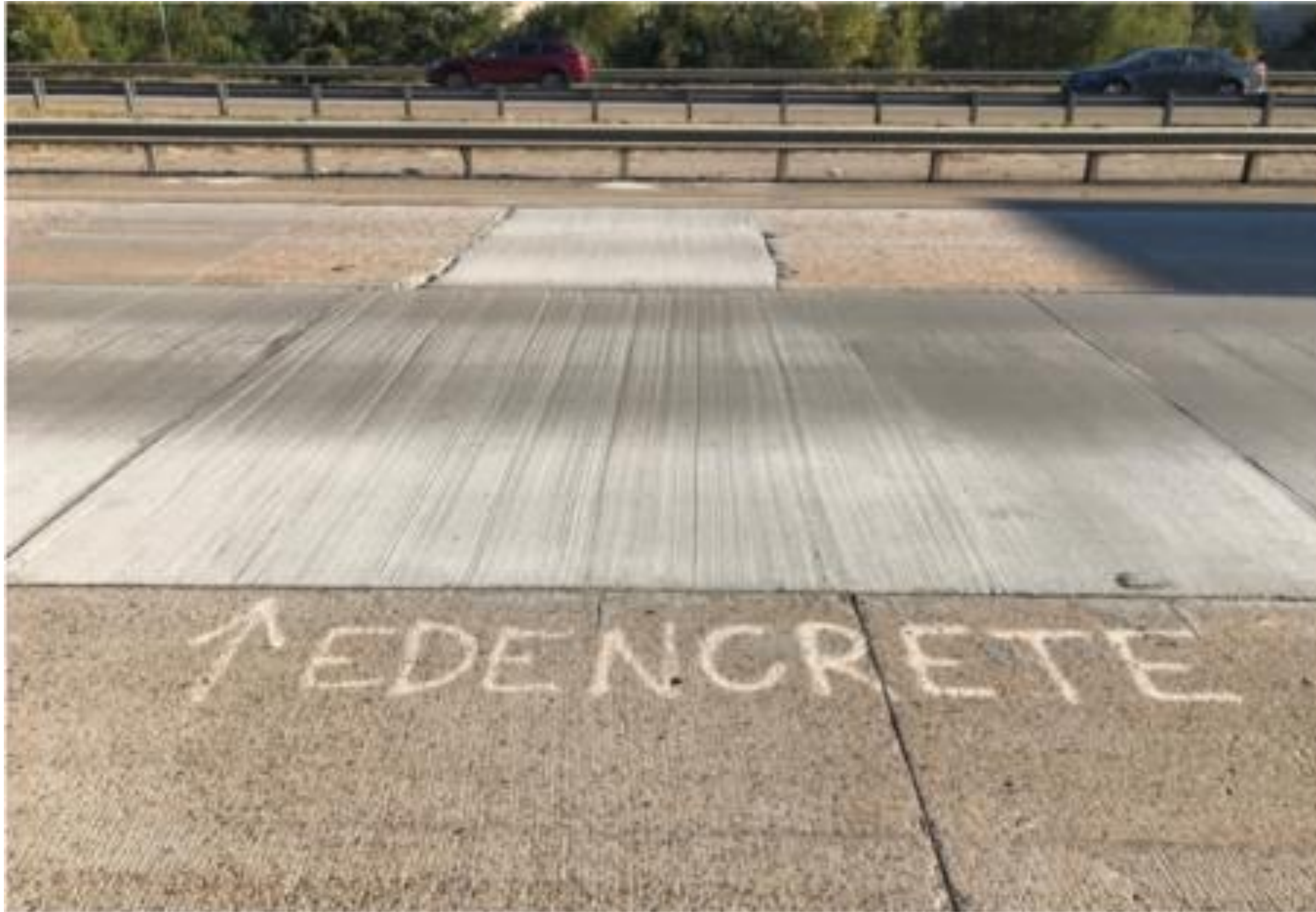
EdenCrete® – No visible cracking or wear
