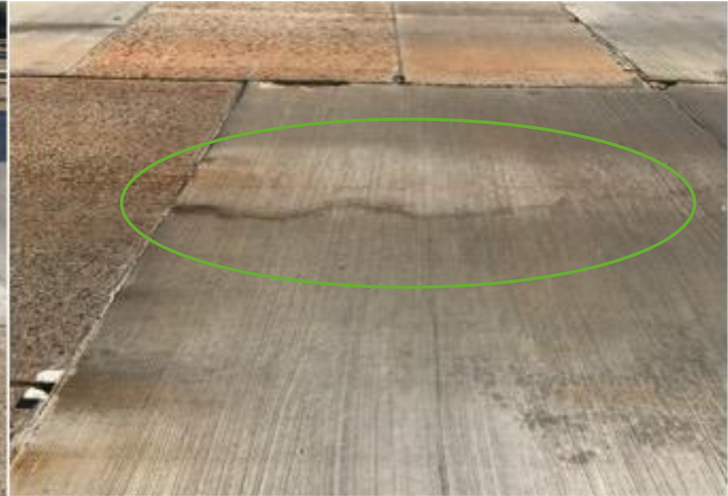
Control – Visible cracking and Wear
