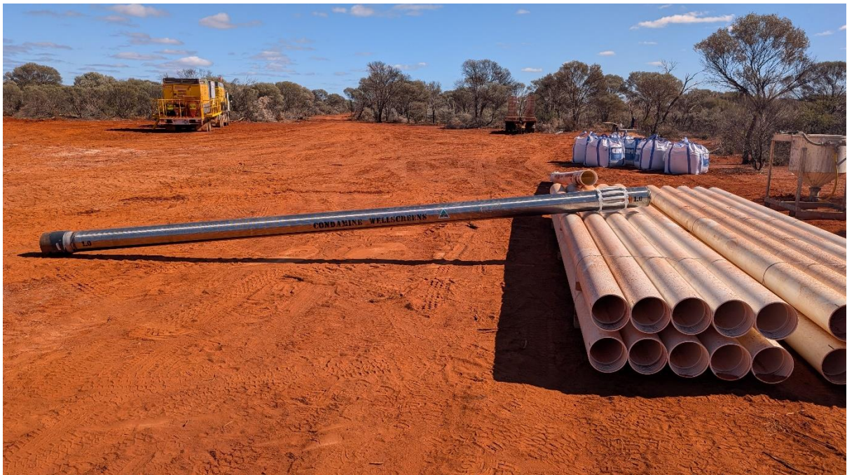
Figure 6 – Screen and casing being prepared for installation
