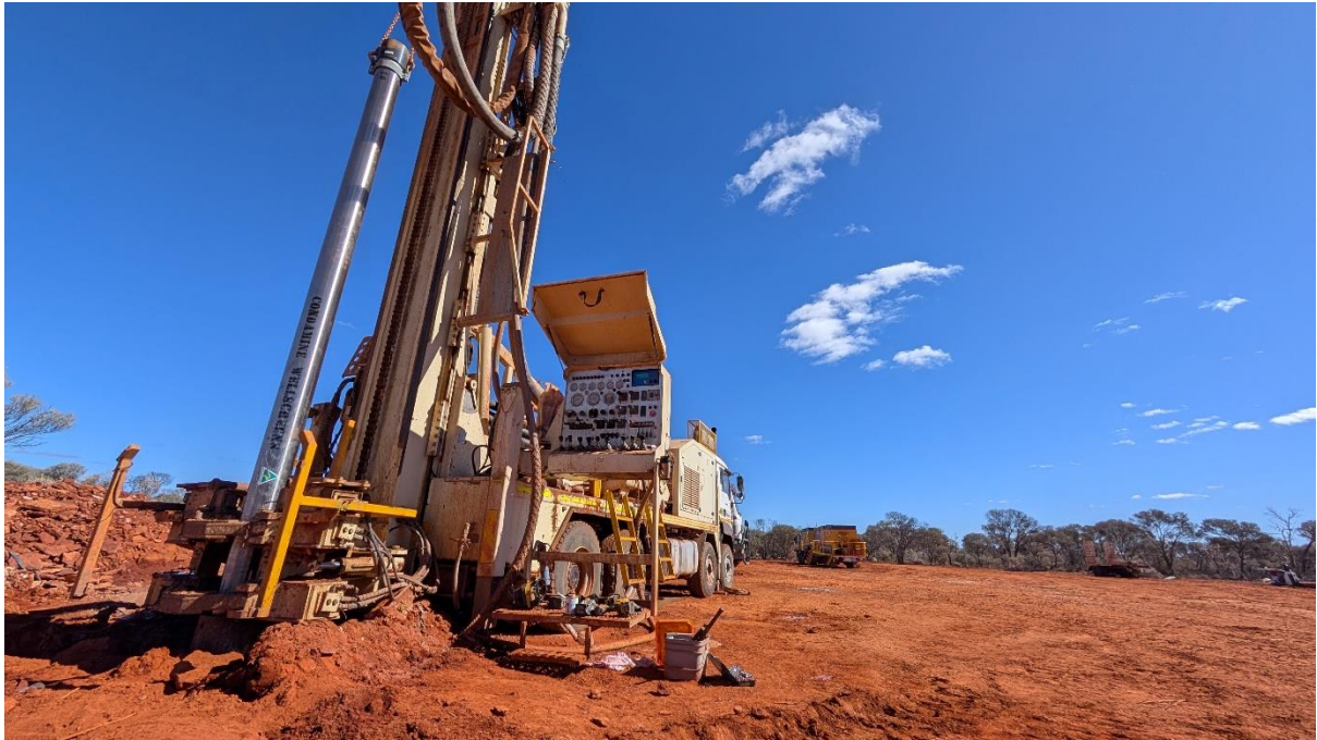
Figure 5 – Installation of bore screen in water production bore
