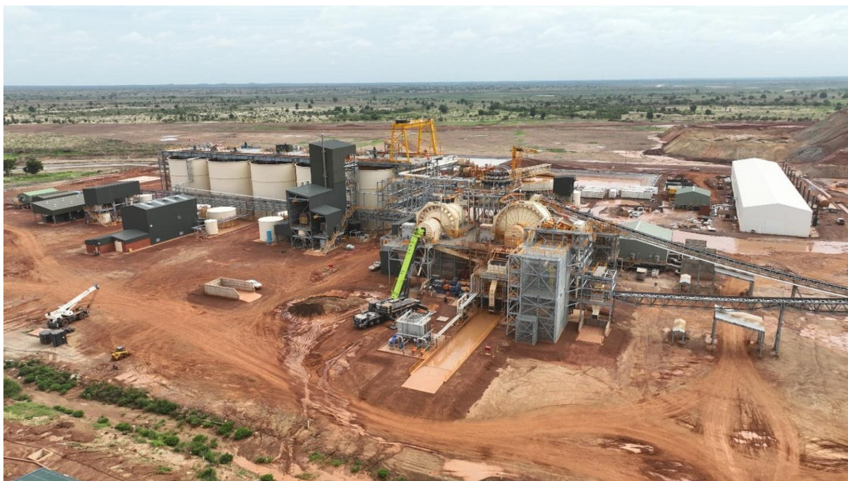
Figure 6 – Kiaka process plant
