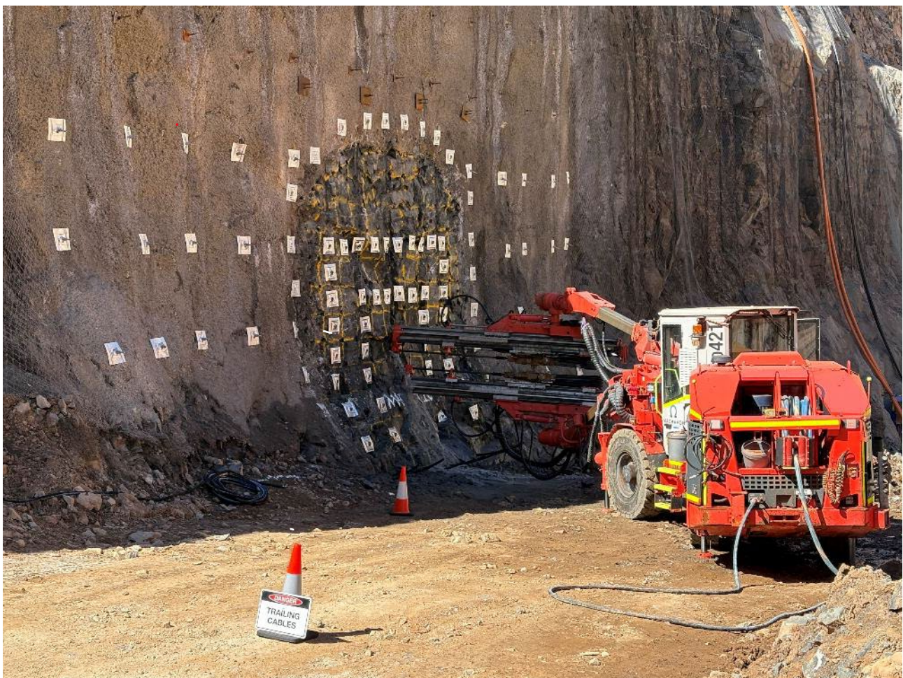
Figure 1: Majestic main decline portal, prior to firing.
