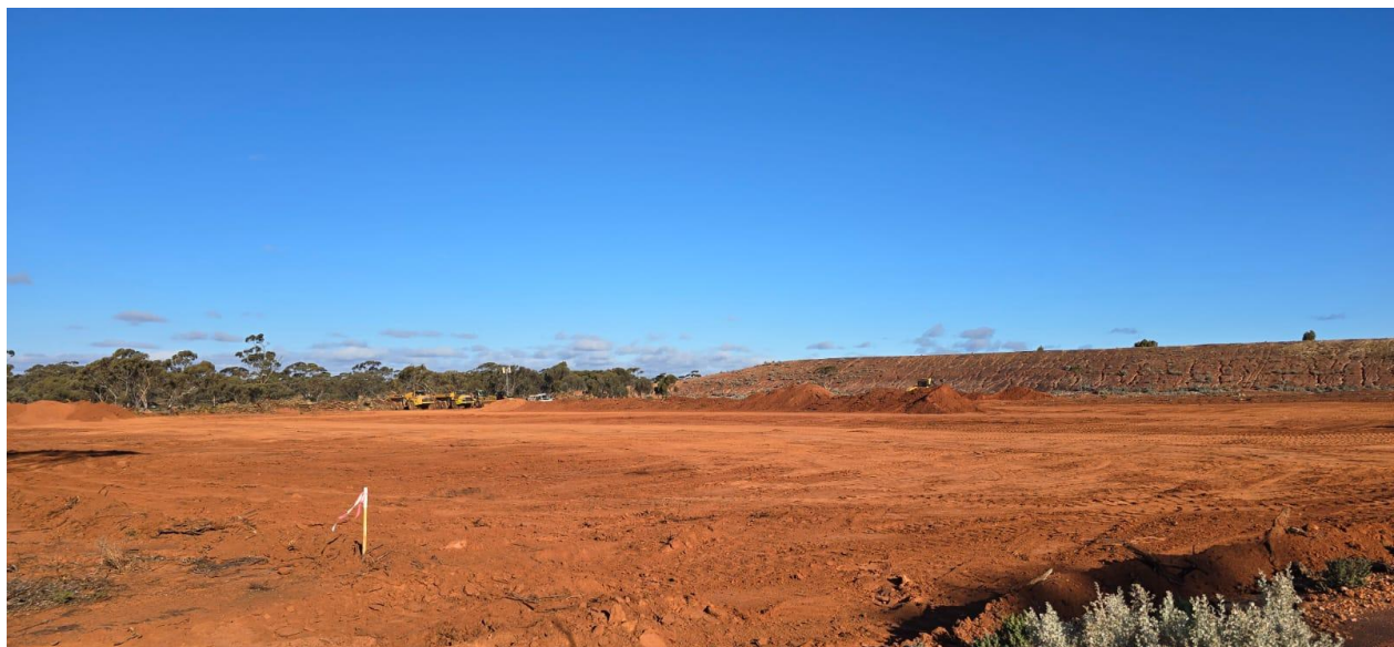
Figure 3: Clearing and topsoil stripping at Fingals workshop/laydown/office area as part of ongoing site establishment activities.
