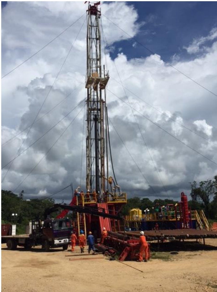
QUN 160 well drilling operations
