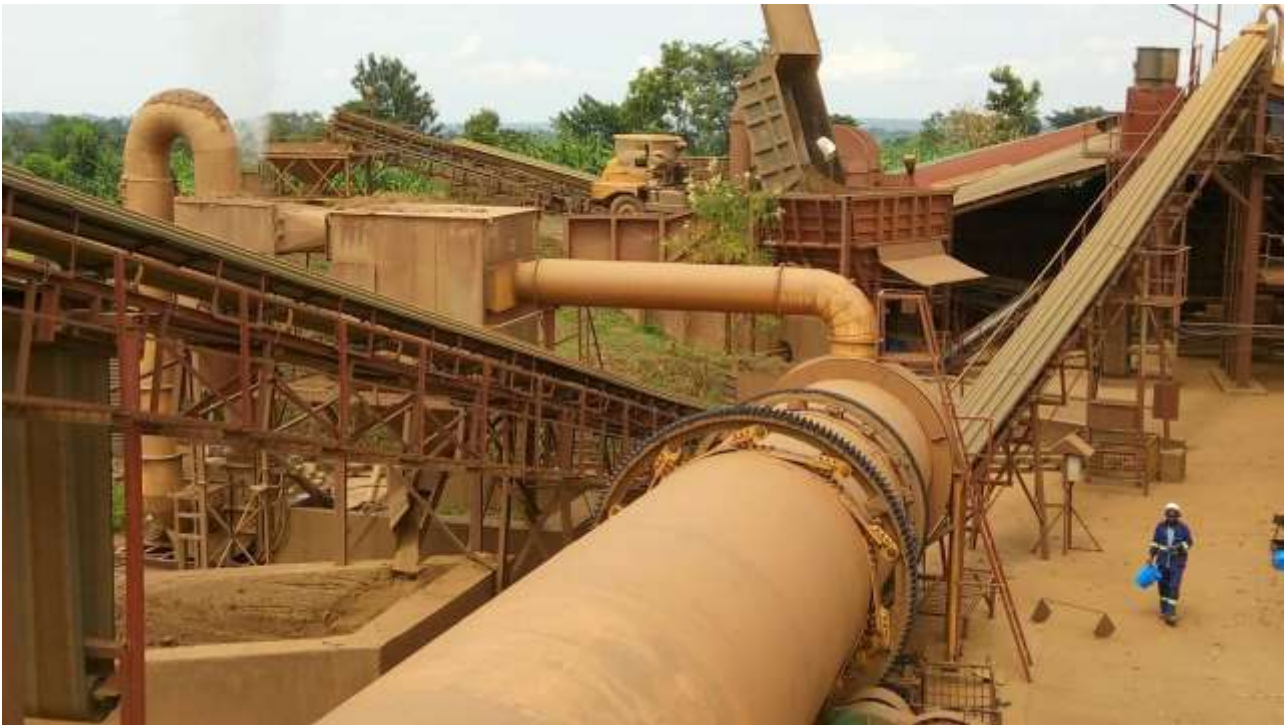
The Namakera Processing Plant - November 2016
