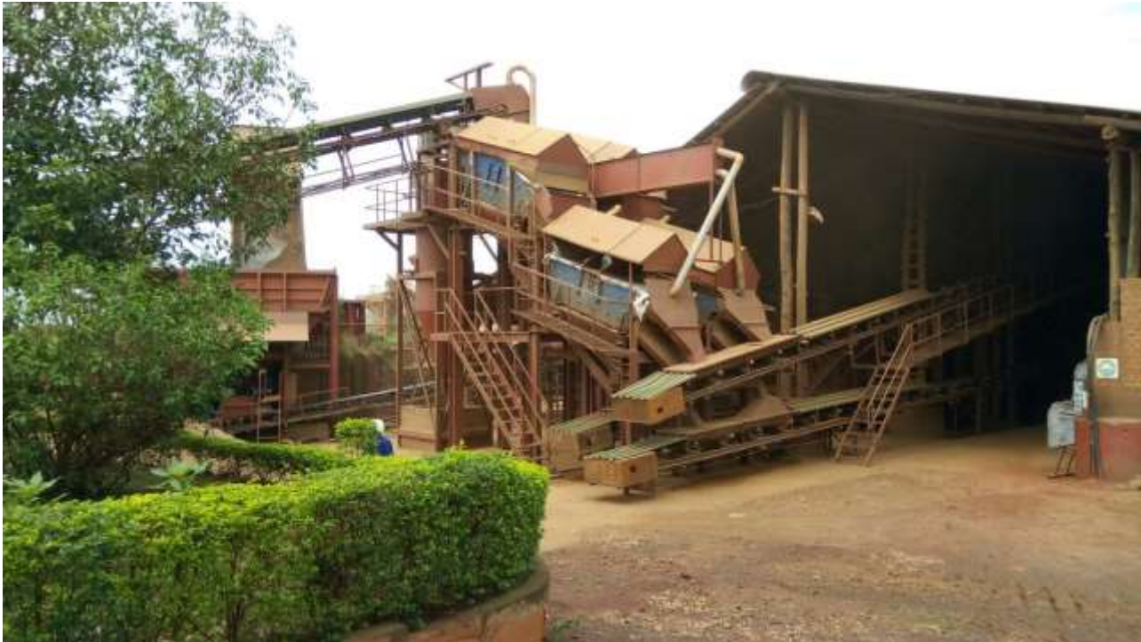
Vermiculite passes through a bank of screens to separate the ore into different size fractions - November 2016
