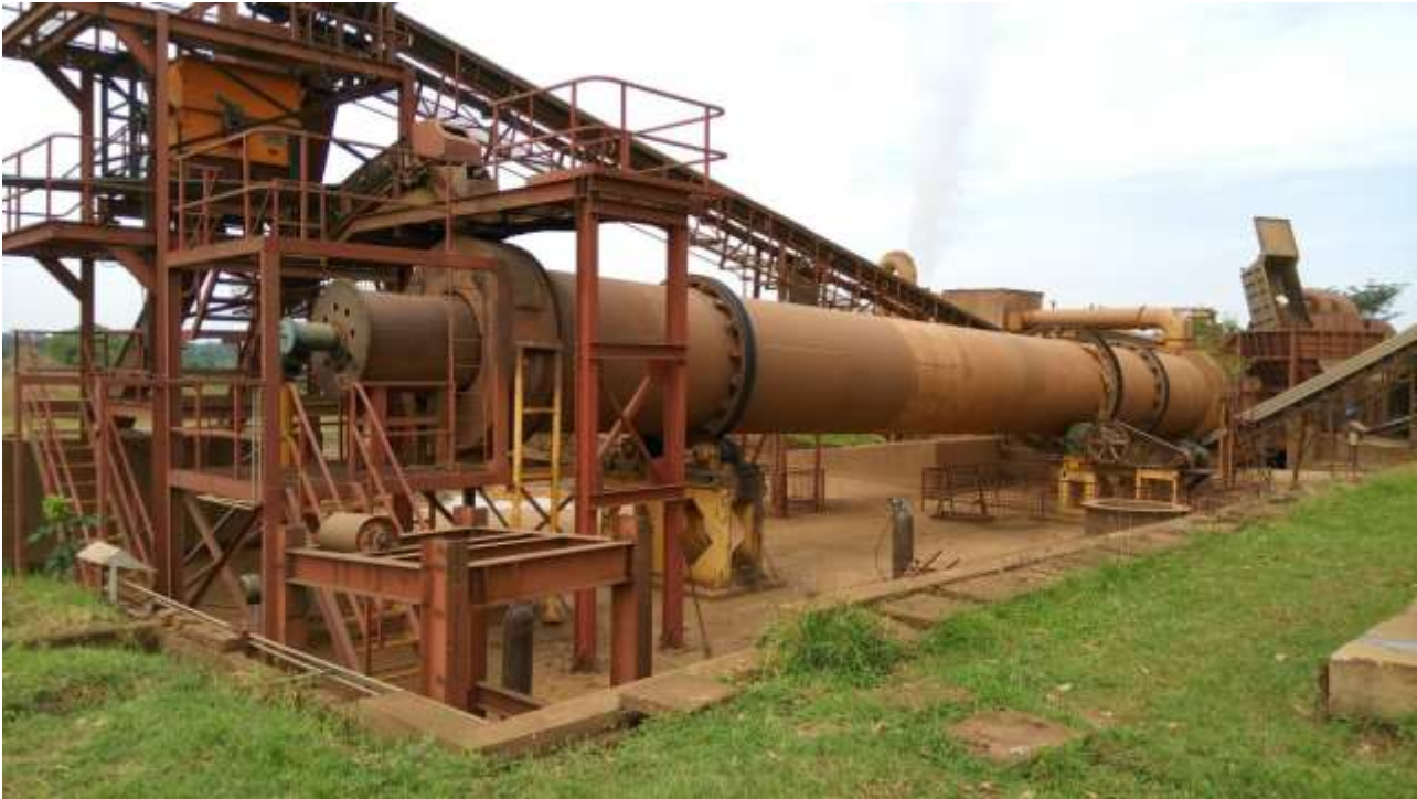
The Namakera Processing Plant with Rotary Dryer centre - November 2016
