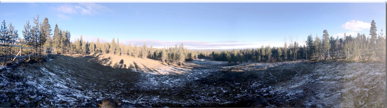
Figure 4 Vittangi open pit has been backfilled and rehabilitation commenced following 2,000m 3 extraction.
