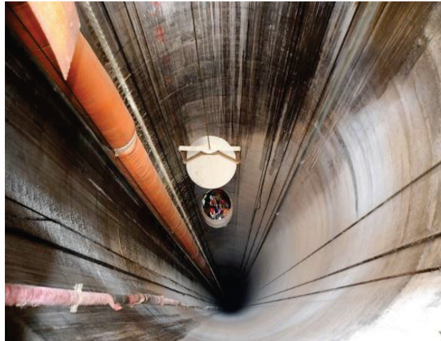
8 Mtpa Coal Mine Shaft - CC5C project utilizing ground freezing
